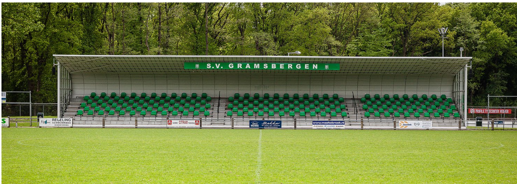
Left The reconstructed stand at SV Gramsbergen ready for another life cycle for its galvanized steel that could reach 100 years in total
